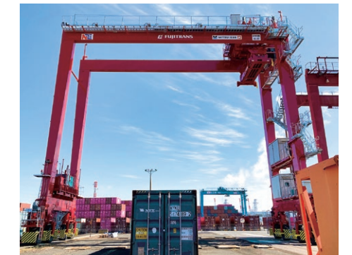
The newly introduced transfer crane
